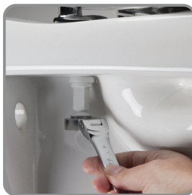
Tighten with Spanner
